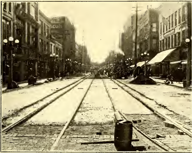
ELMIRA TRACK RECONSTRUCTION—FIG. 11—CONCRETE FOUNDATION, SAND CUSHION AND SPECIAL FILLER PAVING BLOCKS NEXT TO RAILS ON INSIDE OF TRACK
